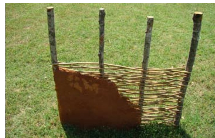
(ABOVE) WATTLE & DAUB STRUCTURE UNDER CONSTRUCTION. (BELOW) EXAMPLE OF WATTLE & DAUB CONSTRUCTION.
