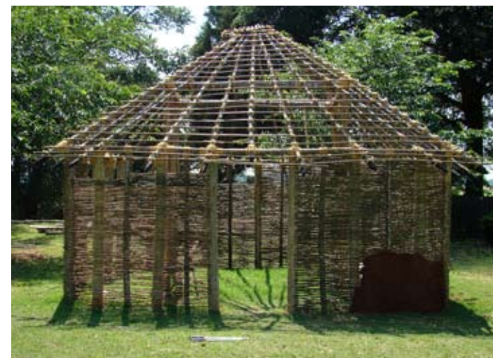
(ABOVE) WATTLE & DAUB STRUCTURE UNDER CONSTRUCTION. (BELOW) EXAMPLE OF WATTLE & DAUB CONSTRUCTION.
